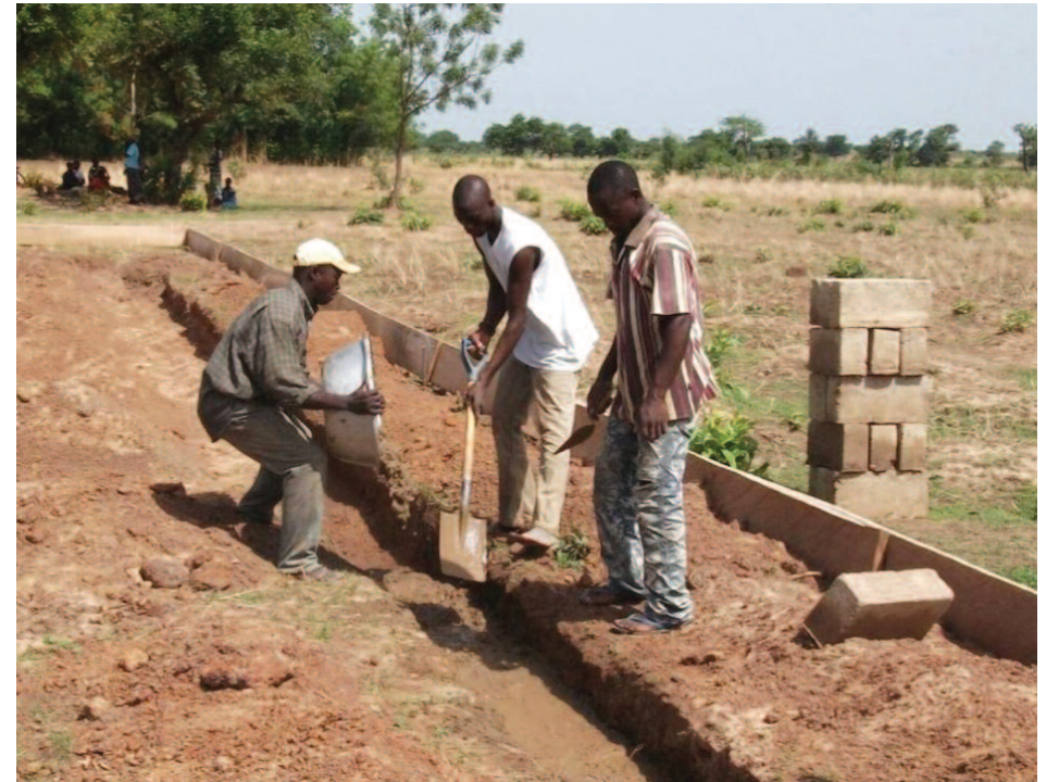
Clearing the land and laying the foundations.
